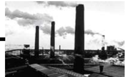
Eskom Coal Based Electricity
