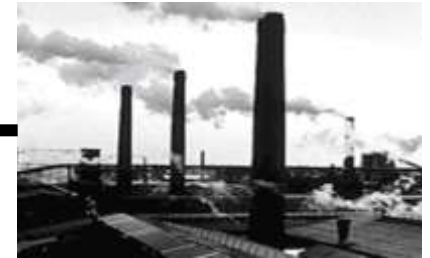
Eskom Coal Based Electricity
